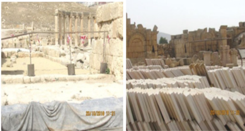
Figure 5: Maintenance at the Temple of Zeus without Posting a Warning Sign
