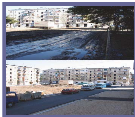
Photo 1: Views from the street rehabilitations in Borough 11
